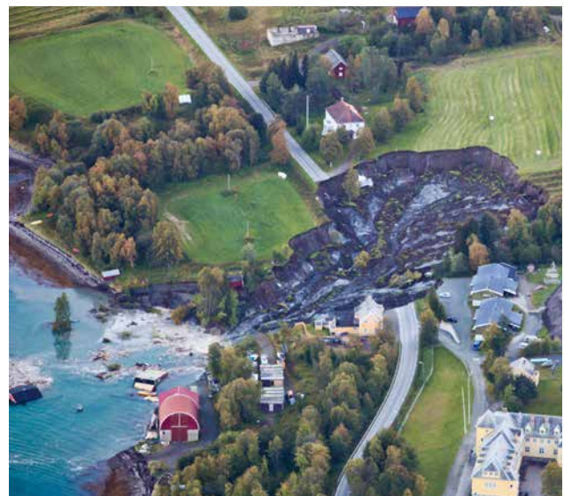
FIGURE 12. Quick clay landslide in Lyngen, September 2010 Photo: Marius Fiskum
